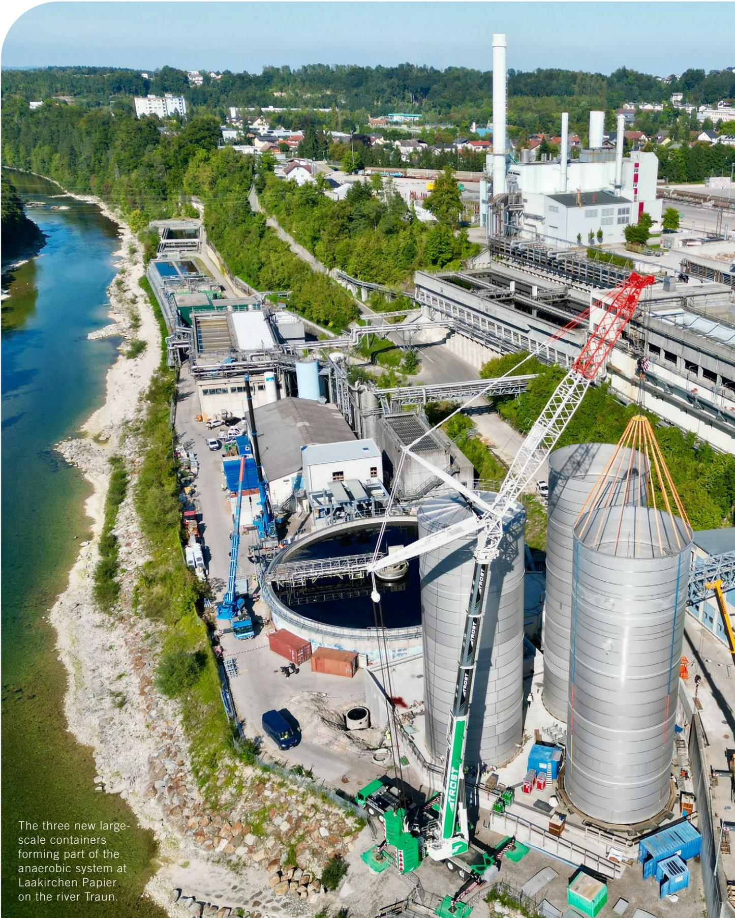
The three new large-scale containers forming part of the anaerobic system at Laakirchen Papier on the river Traun.
