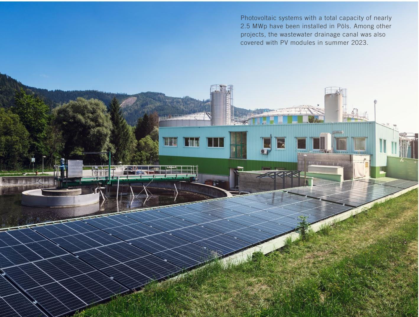
Photovoltaic systems with a total capacity of nearly 2.5 MWp have been installed in Pöls. Among other projects, the wastewater drainage canal was also covered with PV modules in summer 2023.
